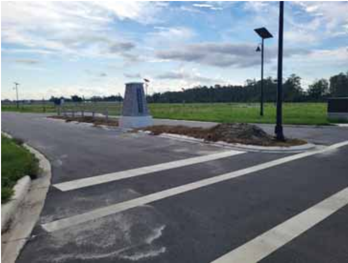
Location 13: Center Island not completed.
